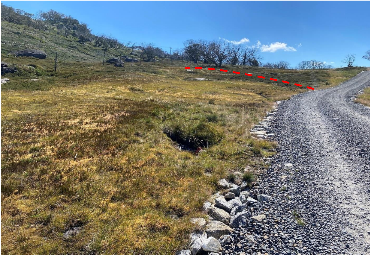
Photo 5: Temporary construction access using a rubber mat to minimise impacts on vegetation will provide access from the Leichhardt access road to the proposed Tower 2.
